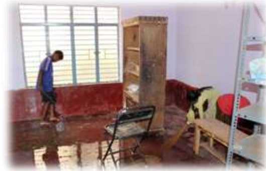
Whitewashing and cleaning of rooms
